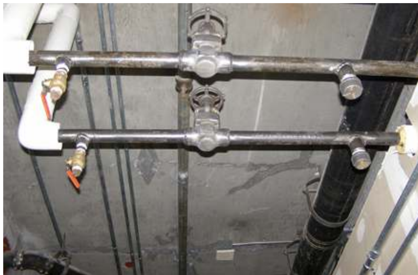
Job Complete with C/S Weld-on Style fittings cap and plug
