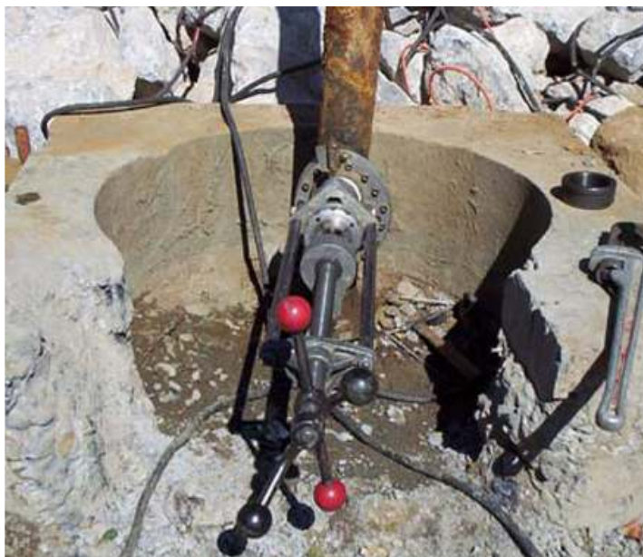
Another Qualitech Line Stop w/ Weld-on Fitting
