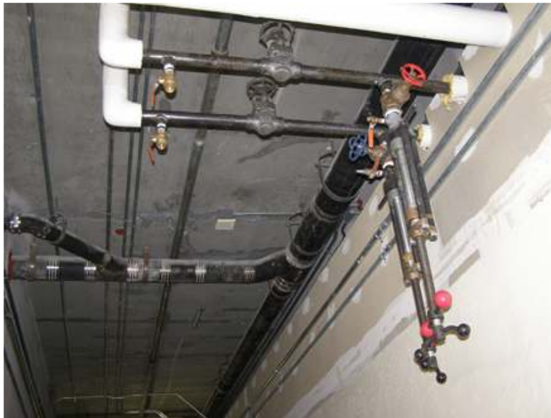
Two Qualitech 1-1/4" Line Stop machine in action
